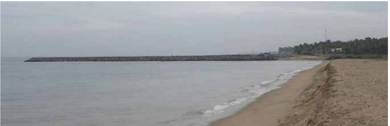
Figure 5.22: May 2007: the last groyne, the largest one - about 170 m long – was built to the north of Thandirayankuppam.
