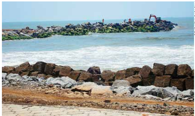
Figure 5.2: Groyne under construction and a seawall along the Malabar coast
